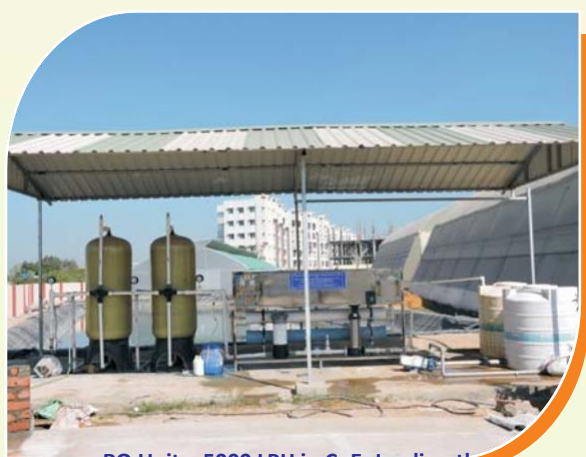
RO Unit – 5000 LPH in CoE, Jeedimetla
